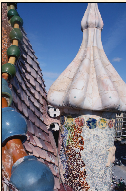
Above: View of the Casa Batlló rooftop
