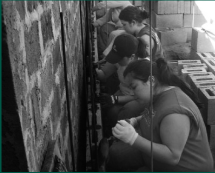
Laying the cement blocks for the Habitat for Humanity house, 2010. (Photo by Natalia Amaya)
